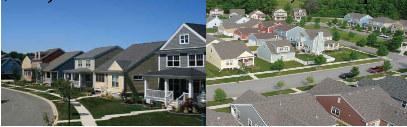
Similar development in The Village in Burns Harbo, Valparaiso, IN. Courtesy of GreenBuilder.
